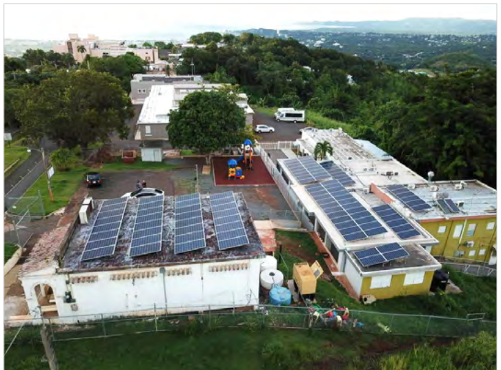
Solar panels charge batteries to store renewable backup power. A generator located between the buildings is used for extended outages.
