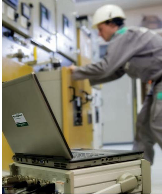
OnSite ProDiag Trip Unit diagnoses trip units on de-energized low voltage circuit breakers
