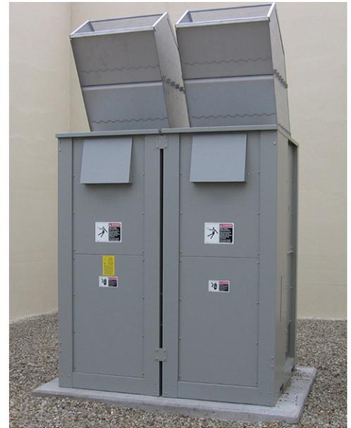
Figure 3: A freestanding load bank with vertical discharge installed on a concrete pad.
