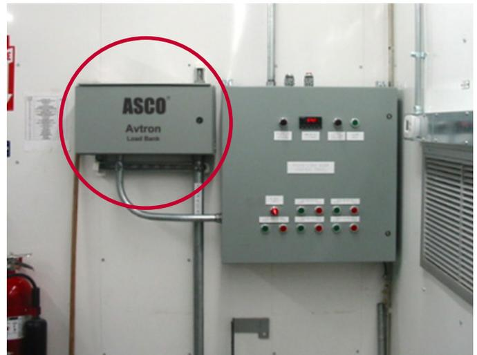
Figure 6: Load Bank remote control panel.
