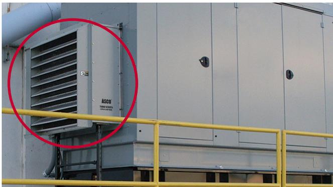
Figure 4: Radiator-mounted load bank with horizontal discharge.
