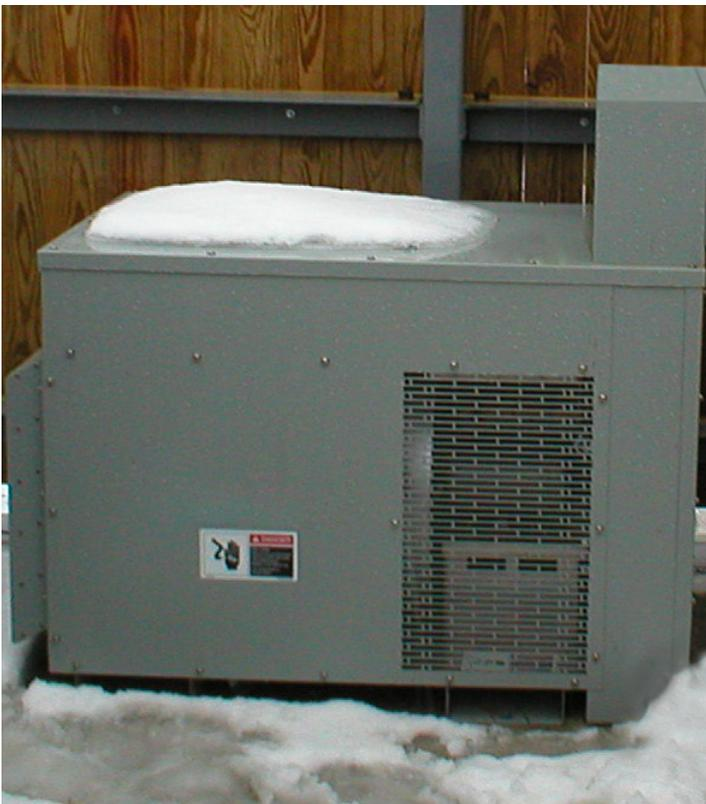
Figure 2: A 150 kW resistive, pad-mounted load bank.
