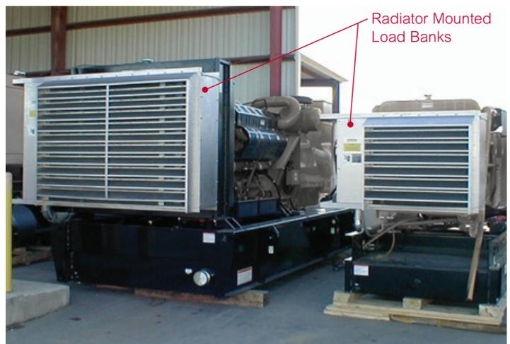
**FIGURE 2:** These diesel gen-sets use radiator mounted load banks to apply the required amounts of load.
