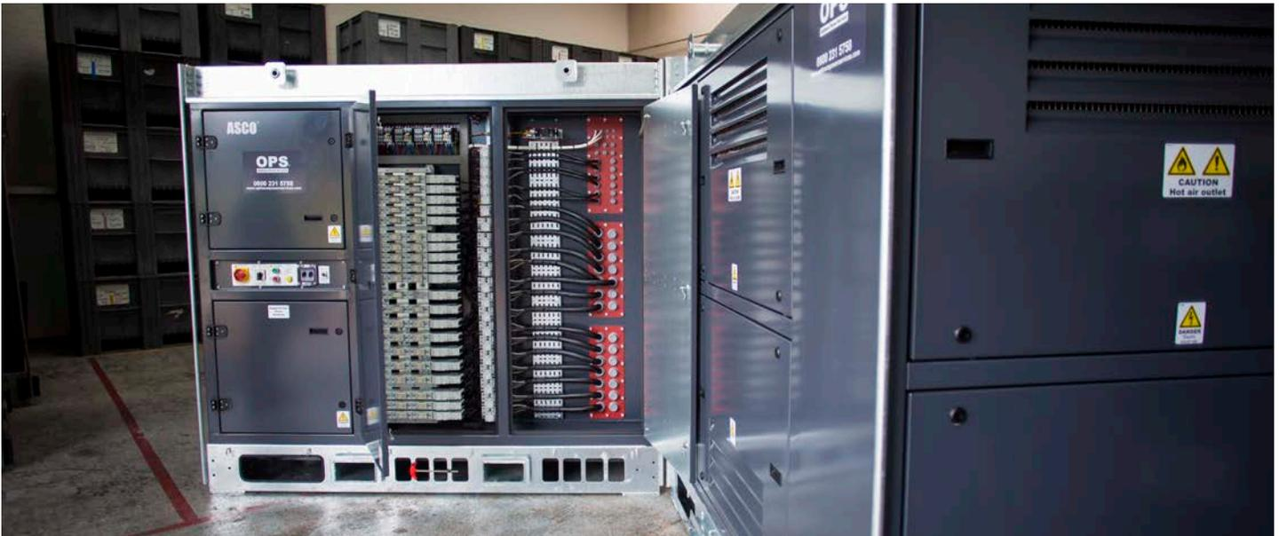
**Figure 3:** A 600 kVAr Capacitive Load Bank. Photo courtesy of Optimum Power Services.
