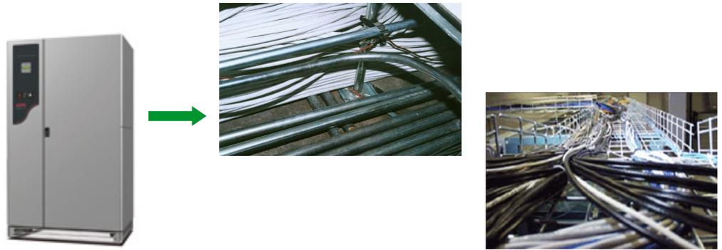
The electrical contractor plays a large role in engineering this type of solution and a significant amount of wiring work is done onsite, including cutting, terminating, and connecting each individual branch circuit, and routing them to the racks. In a raised floor installation, special under-floor mounting supports are engineered as well. For branch level metering, sensors are added and then programmed.
