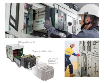
Illustration of an aging, obsolete circuit breaker replaced by a modern circuit breaker while maintaining the original cradle.
