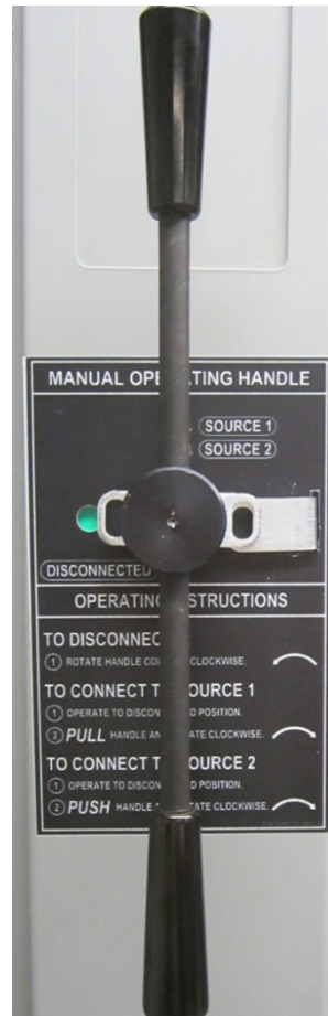
Figure 3. DISCONNECTED (from SOURCE 1 or SOURCE 2) position indicator
