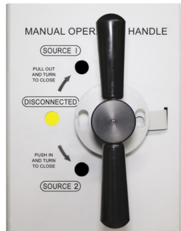
Figure 3. DISCONNECTED (from SOURCE 2) position indicator
