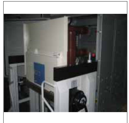
Fig. 6.2 Couple the transport truck to the panel.
