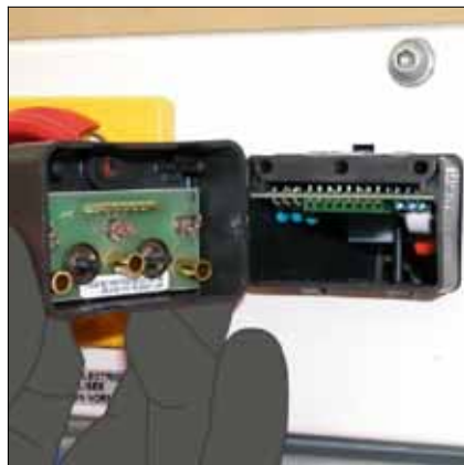
J Extract the voltage indicator unit.
