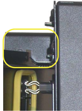
Figure 9: Positioning the Plug-In Unit onto the Busway
