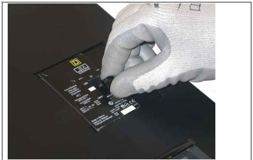
Figure 12: Turning the Plug-In (Tap-Off) Unit to the ON (I) and OFF (O) Positions
