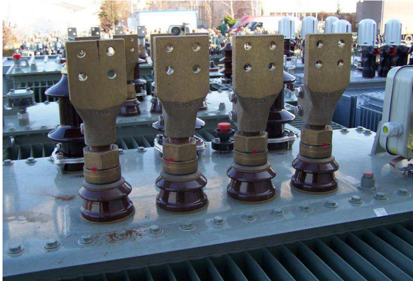
Fig. 7. LV bushings according to DIN 42530 or EN 50386:2010 with flat terminals.
