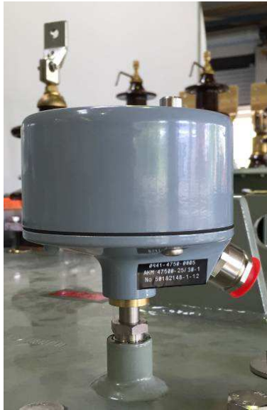
Fig. 18. Pressure sensor - AKM type.
