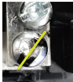
Figure 15 – Apply Mark after Tightening Right Bottom Neutral Bar Screw
