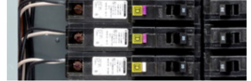
Plug-on Neutral connection
