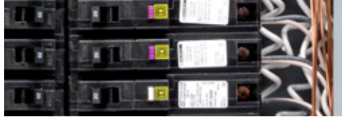
Pigtail neutral connection
