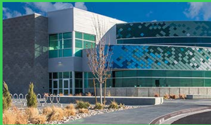
Modernizing a 100-year-old school
