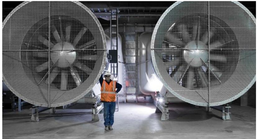
system adjusts the VSD on each operating fan to ensure fan operation is fine-tuned according to conditions.
