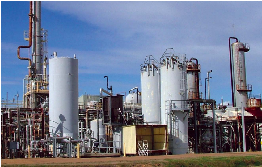
Foxboro Conductivity Sensing Sparks Automated, Efficient Biodiesel Fuel Processing
