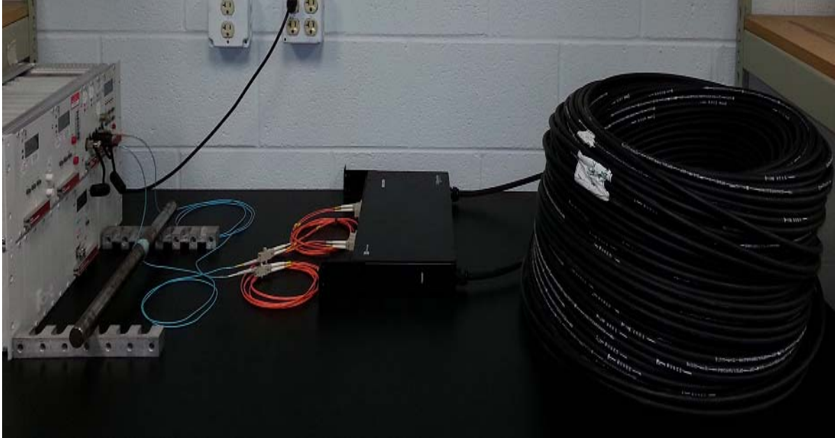
Figure 4: 6 Channel Link System MM (OM3) Configuration Test Setup
