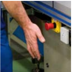
Example of applications: Resetting following activation of an emergency stop.
