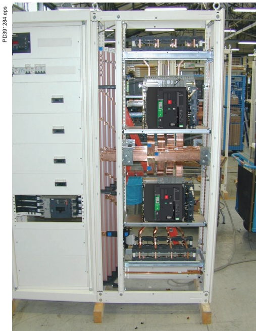
Source changeover system in 2 combined cubicles.
