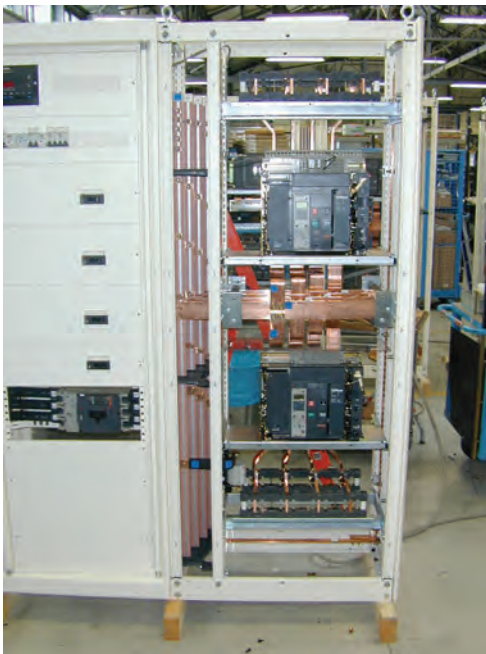
Source changeover system in 2 combined cubicles.
