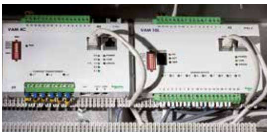
The arc sensor I/O units incorporate a snap-in connector for the portable sensor. The activated arc sensor channel is indicated with a led.
