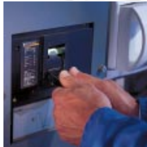
Switching on incoming circuit-breaker
