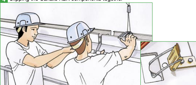
4 Clipping the Canalis KBX components together
