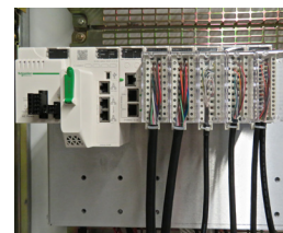
PLC-5 I/O quick wiring adapters mounted on an M580 PLC
