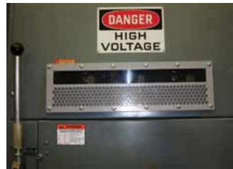
CAP-V24 installed on Square D HVL
