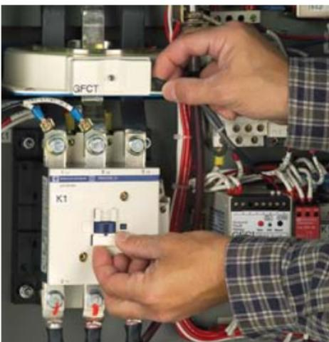
New Article 409 covers industrial control panels that are intended for general use and operate at a voltage of 600V or less. In addition, this article recognizes in Table 409.3 that industrial control panels may be constructed and
