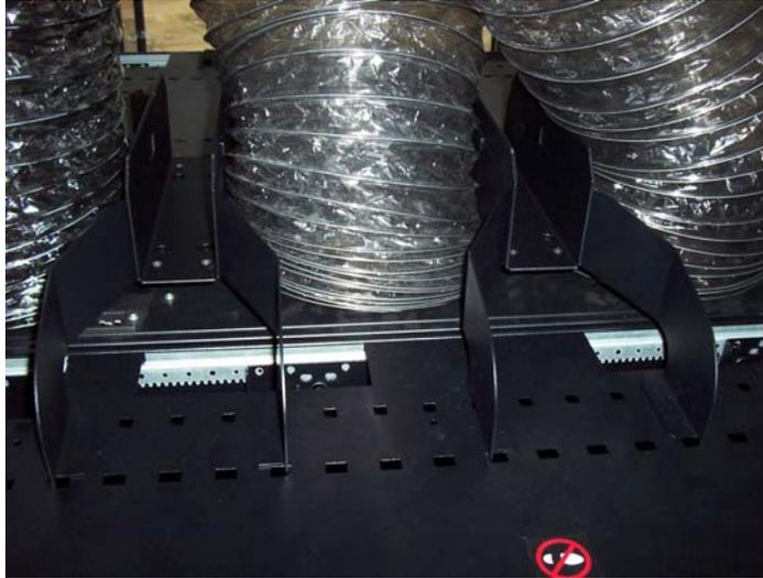
Figure 7 – InRow SC with cable support bridge troughs in “non-bridge” application
