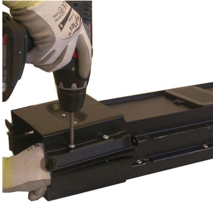
Figure 16: Installing Flange Screws on Clamping Brackets
