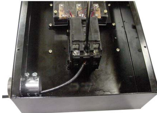
Figure 16: Tap Box Wiring
