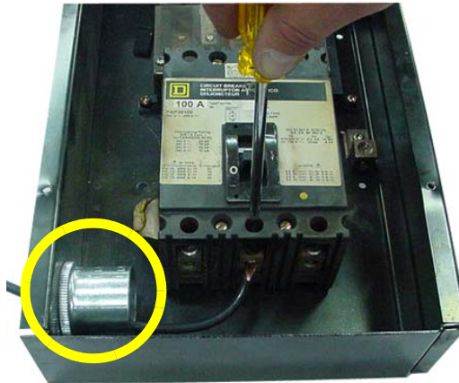
Figure 14: FA Load Side Wiring
