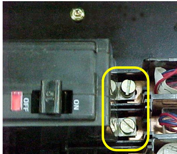
Figure 31: QOB Line Side Connection
