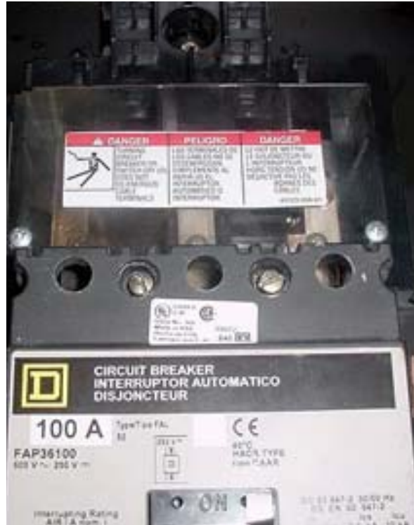
Figure 4: Reverse Feed Label Placement (Circuit Breaker)
