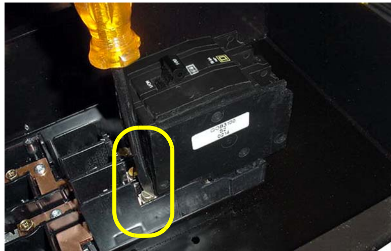
Figure 40: Removing the QOB Circuit Breaker
