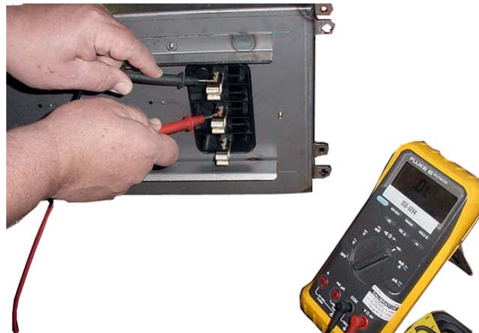
Figure 7: Testing Plug-in Unit Isolation Prior to Installation
