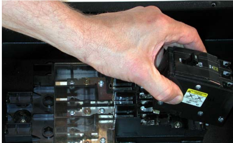
Figure 28: QO Circuit Breaker Installation
