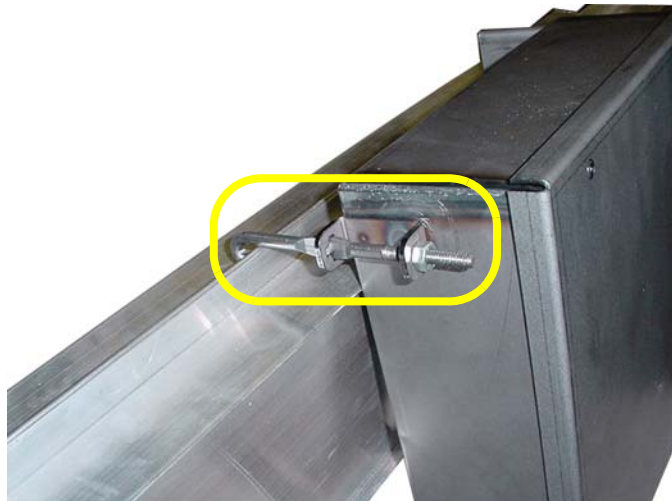
Figure 13: Securing the Plug-in Unit Onto the Busway
