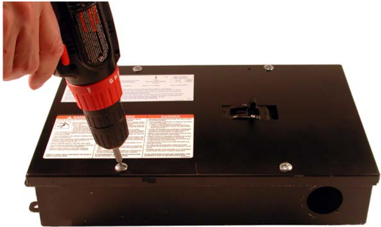
Figure 38: Remove the Enclosure Cover
