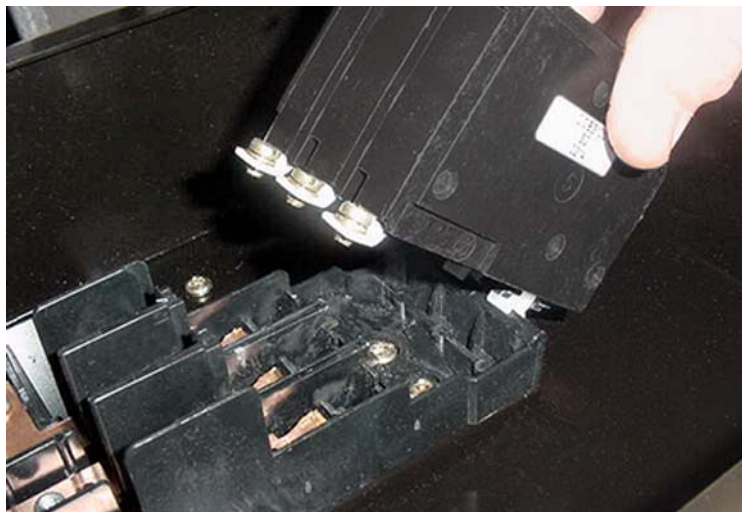
Figure 41: Removing the QO/QOB Circuit Breaker
