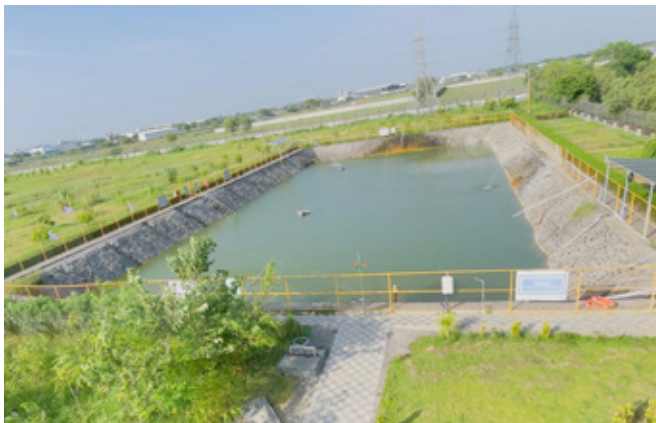
Rainwater Harvesting Pond at MVI Vadodara
