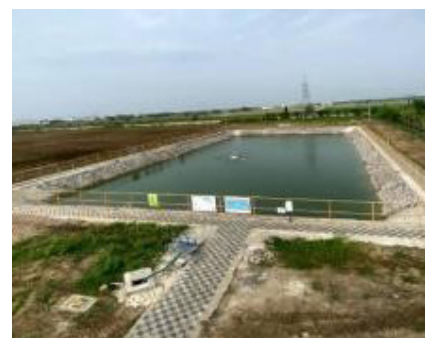
➤ Rain water Harvesting pond at MVI Baroda
