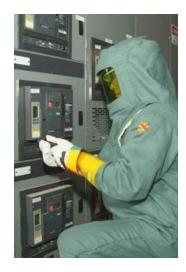
To help mitigate arc flash risk, it is important to perform an investigation that assesses a worker's potential exposure to arc flash energy. That is conducted for the purposes of injury prevention, determination of safe work practices, and appropriate levels of personal protective equipment (PPE). The general process of conducting such an assessment follows these steps:
