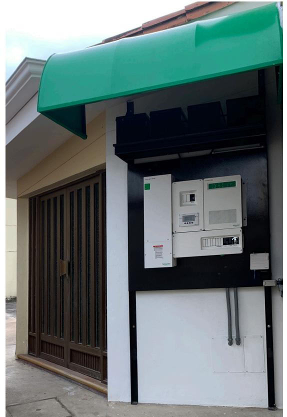
HMB Solar designed 4 kW DC-Coupled grid-interactive system
