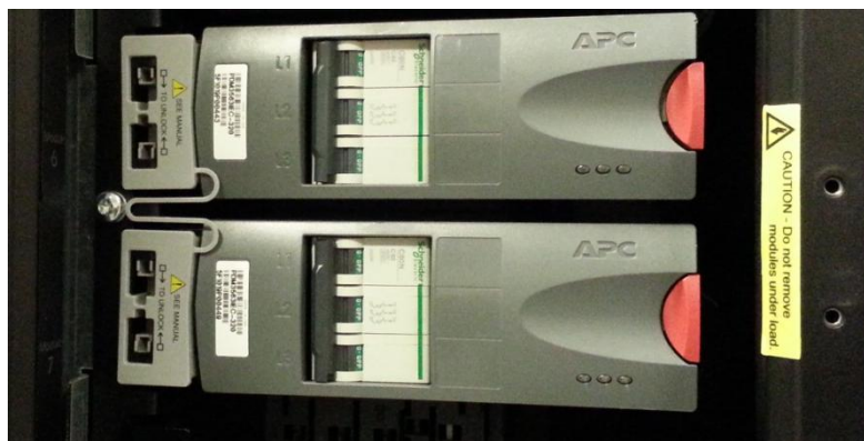
Figure 1: Slot locks installed near the Power Distribution Module hinges to block insertion or removal of PDMs
