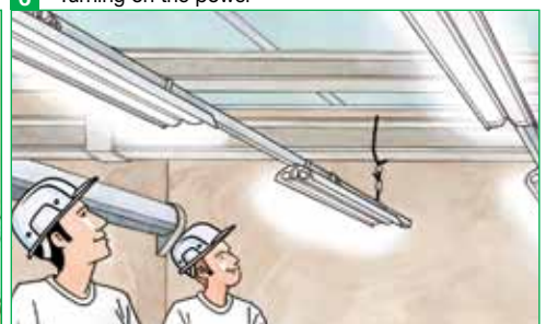
6 Turning on the power
