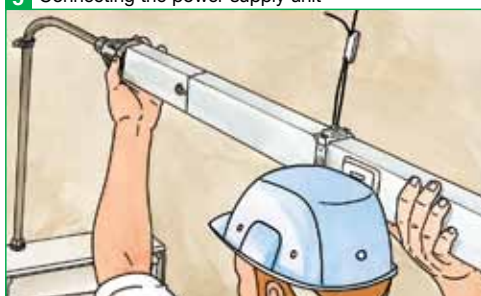
5 Connecting the power supply unit
