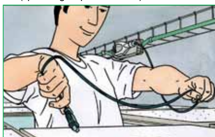
5 Connecting the lights (up to 5 lights per connector)
