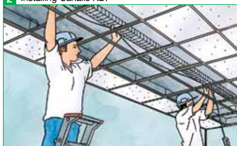
2 Installing Canalis KDP
