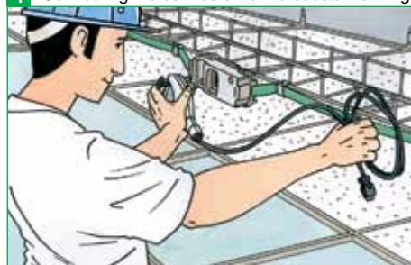
4 Connecting the connector to the busbar trunking
