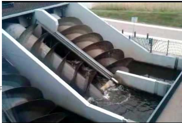
Sludge lift in wastewater
