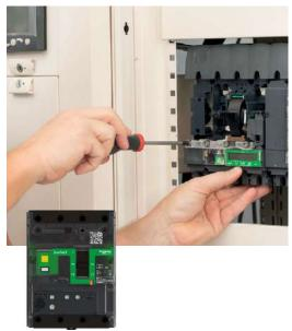
Integrated earth leakage protection
