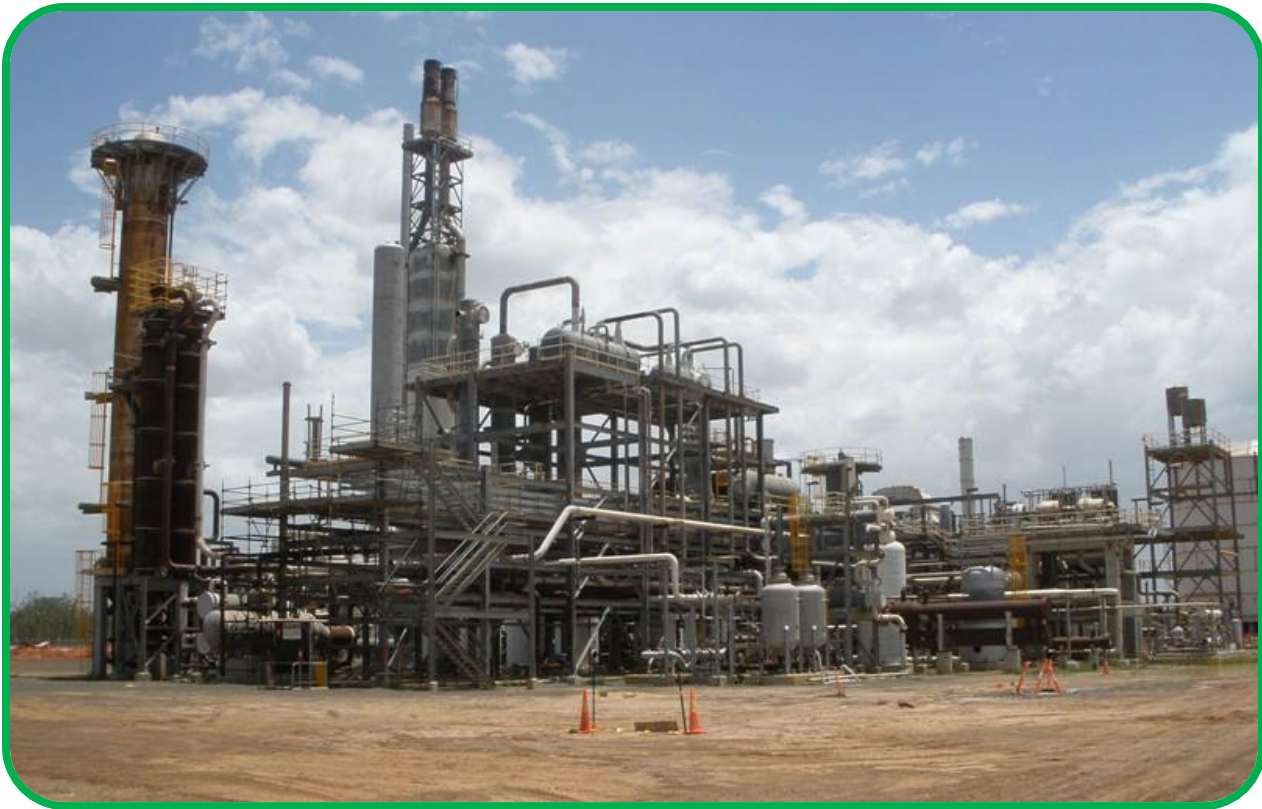
A specialty chemicals plant
