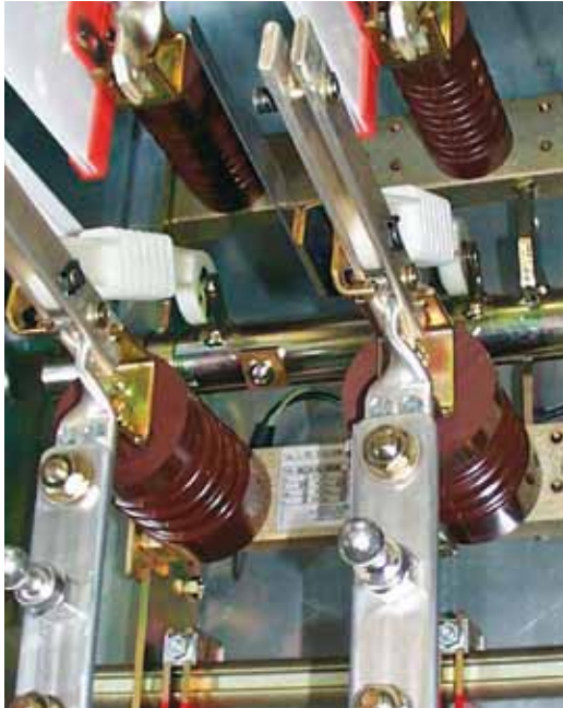
Divider attachment on the moving-contact side
