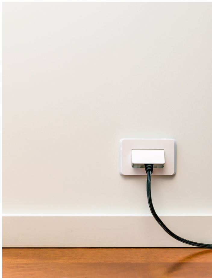
Aesthetically appealing cable management
