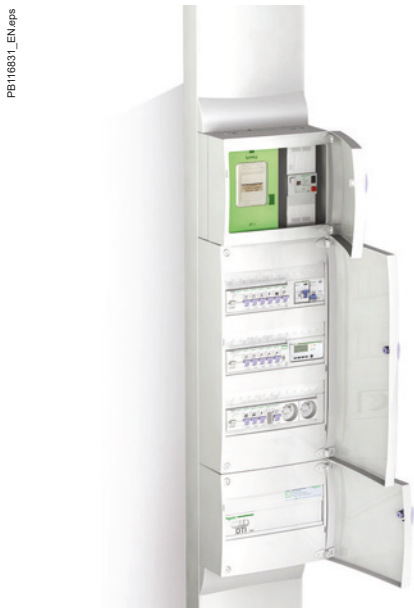
Fig. Q6 Example of control and distribution board (France)
