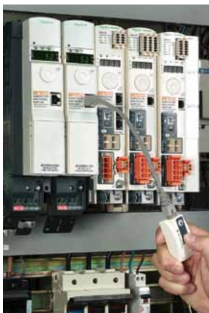
Simple-Loader: duplicates a configuration on two identical drives
