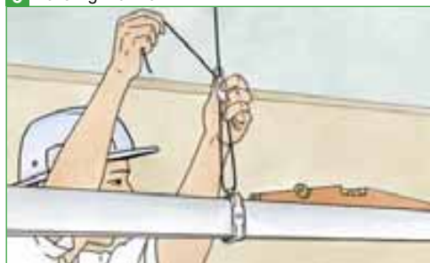
3 Leveling the line
