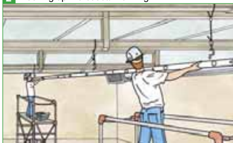
2 Hooking up the busbar trunking
