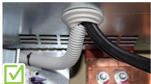
Cable glands are used to protect cables from the hole in the sheet.
