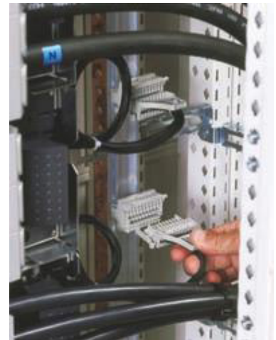
Auxiliary connection block in the connection compartment.
