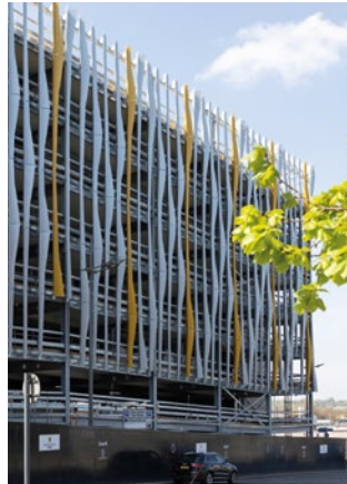
Multi-storey car park
